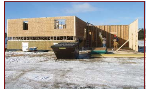
House under construction in Bemidji
