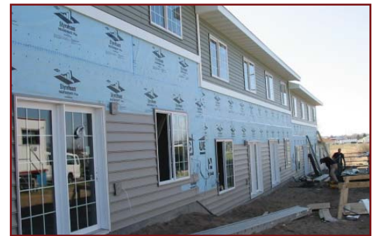
Siding installation on 8-plex in Detroit Lakes
